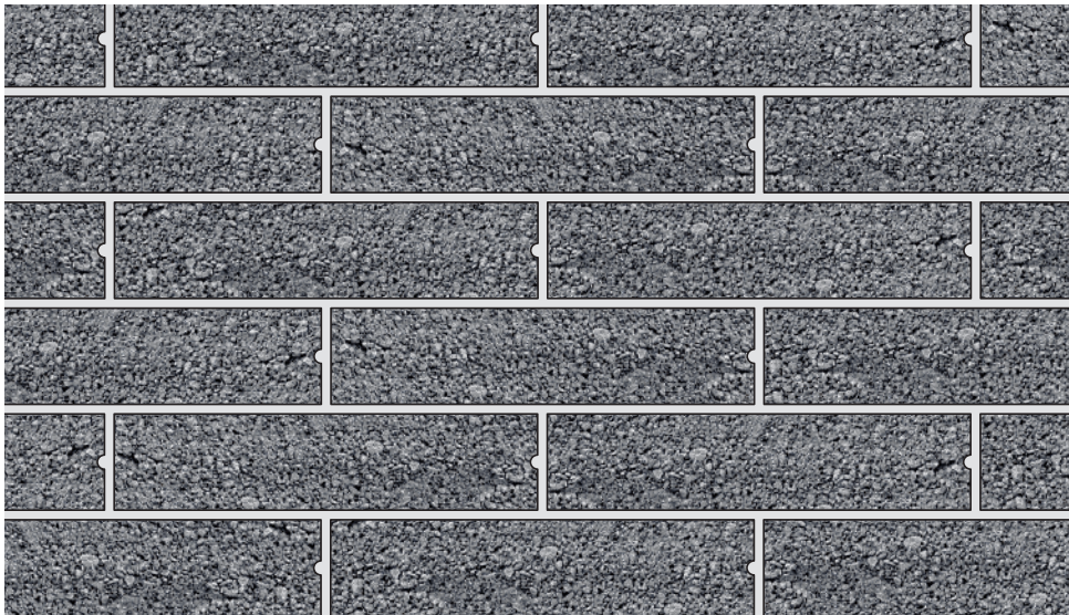
Appearance of Stowells RD separating wall as built
