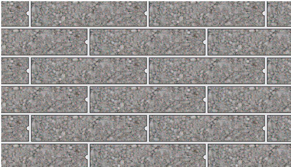
Appearance of PLASCON separating wall as built
