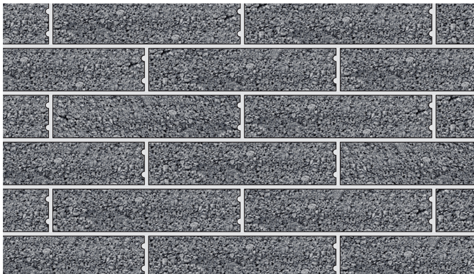
Appearance of Besblock dB Performer separating wall as built
